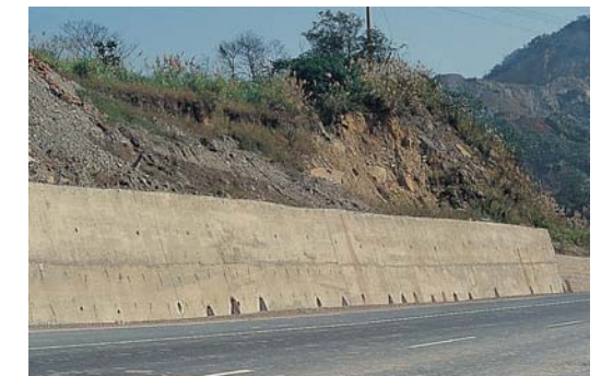
▲ 公路檔土牆 Highway soil bulwark.
